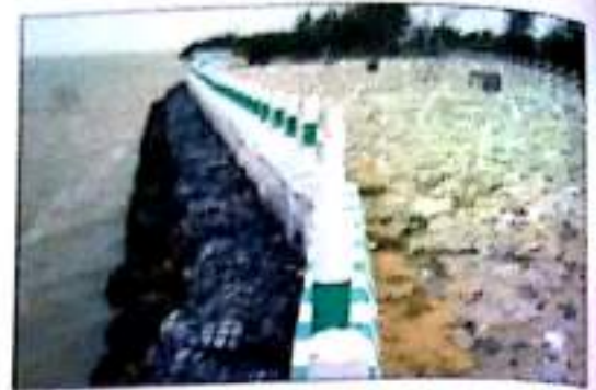
Fig. 11 Protection works against sea erosion at Puri-Konark Road
