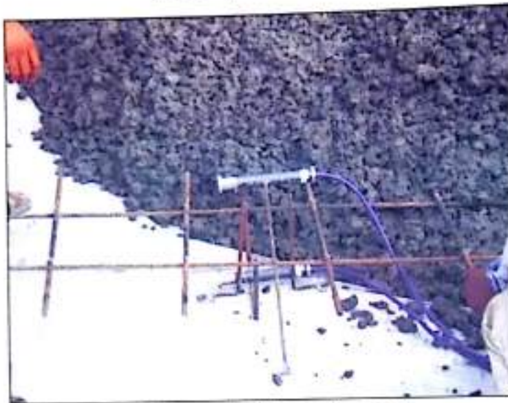
Fig. 39 Sensors embedded in concrete pavement
