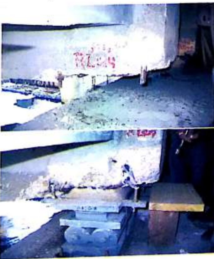
Fig. 76 Replacement of roller bearings
