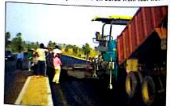
Fig. 29 Laying of plastic waste modified mix at Rohtak-Bhiwani road
