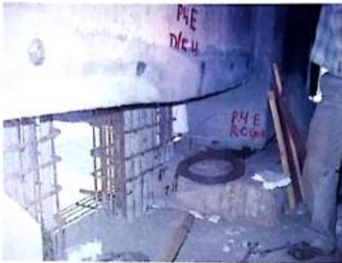
Fig. 77 Reinforcement of seismic restrainer
