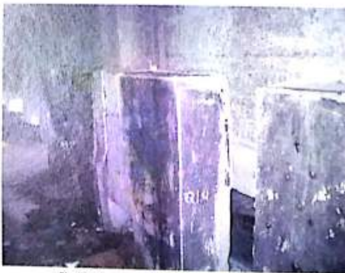
Fig. 78 Neoprene pads provided in seismic restrainers
