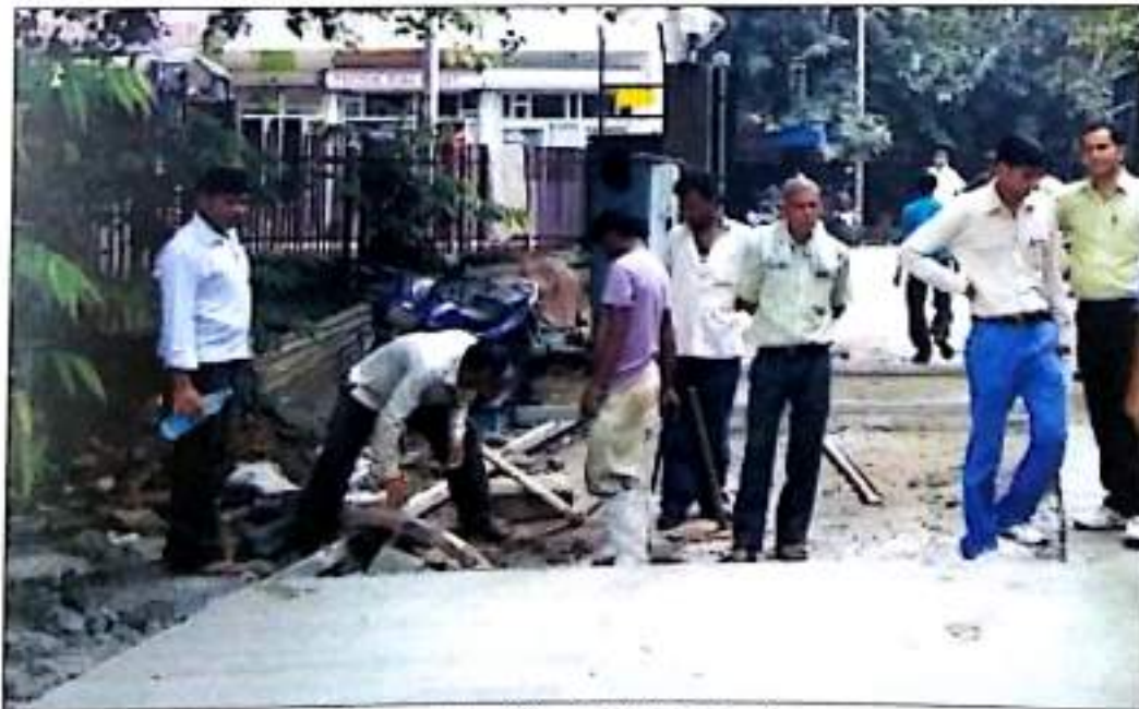
Fig. 43 Construction of Ultra Thin White Topping in progress
