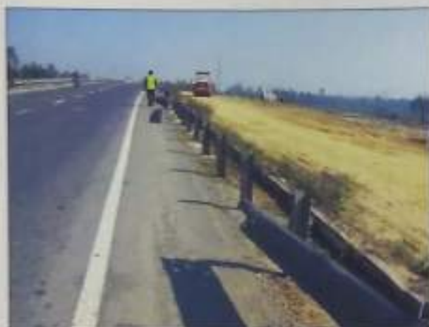
Fig. 98 Damaged crash barrier (w-beam) can be a safety hazard to road user at km 159.760 on Moradabad - Bareilly section of NH-24
