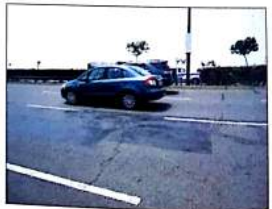
Fig. 56 View of transverse cracking and crack sealing on the main carriageway of DND Flyway (Delhi to Noida)
