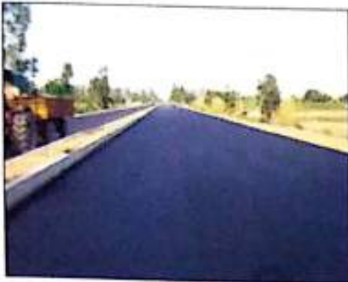
Fig. 30 Finished surface of plastic waste modified mix at Rohtak - Bhiwani road
