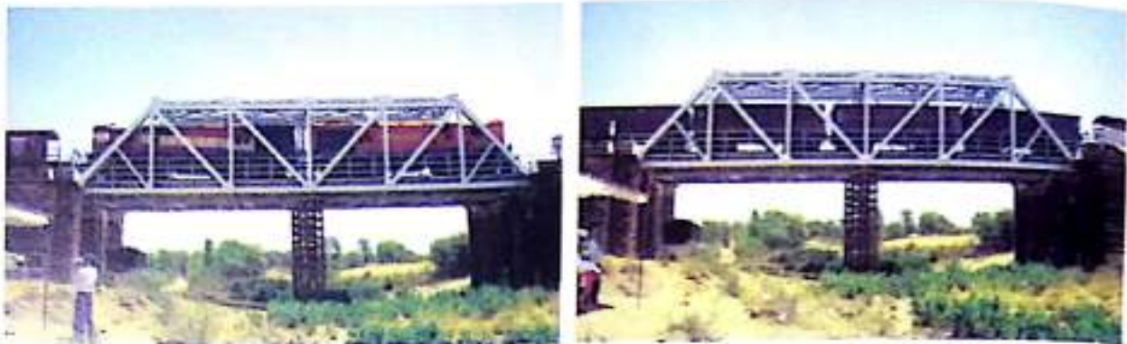
Fig. 73 Test train over the bridge under various loading conditions
