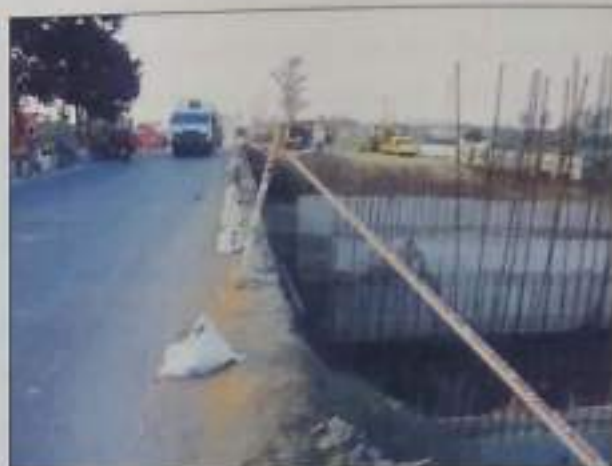
Fig. 99 Inadequate barricading and delineation at km 261.000 on Moradabad - Bareilly section of NH-24
