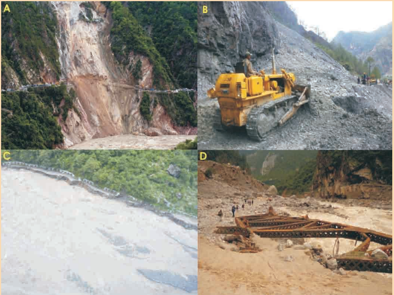
Fig 2: A. Tourists stranded at Kaliasaur landslide & B. BRO workers restored the highway connectivity at Patalganga Rockfall on NH-58 respectively. C. & D. Washed out road formation near Pandukesaur area & Damaged Bridge near lambagarh area due to flash flood in Chamoli district respectively
