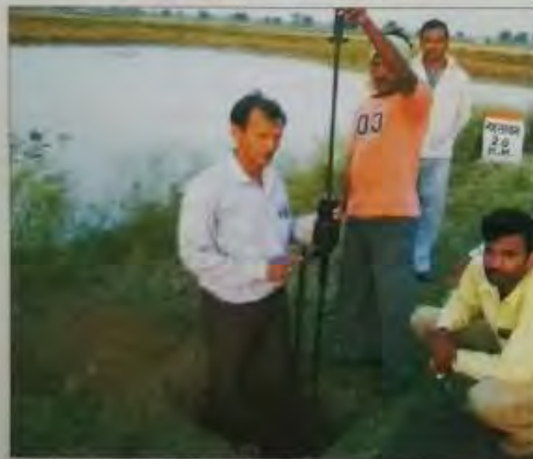
Fig. 8. DCP tests at sub-grade level
