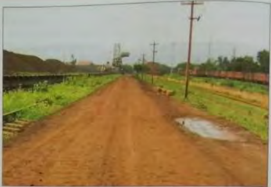
Fig. 32 View of 3rd tippler approach of H2 drive House in DHC along East side of S1 conveyor
