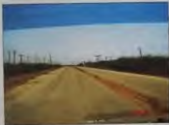
Fig. 60 A view of the DLC laid over the road in Vilayat Industrial Estate
