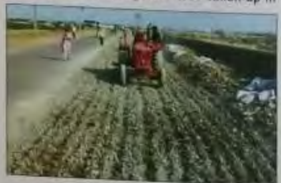
Fig. 20 Cement stabilisation of C&D waste for test road construction
