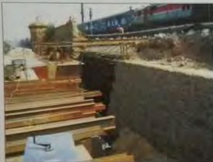
Fig. 11 Trains running smoothly after dismantling of retaining wall
