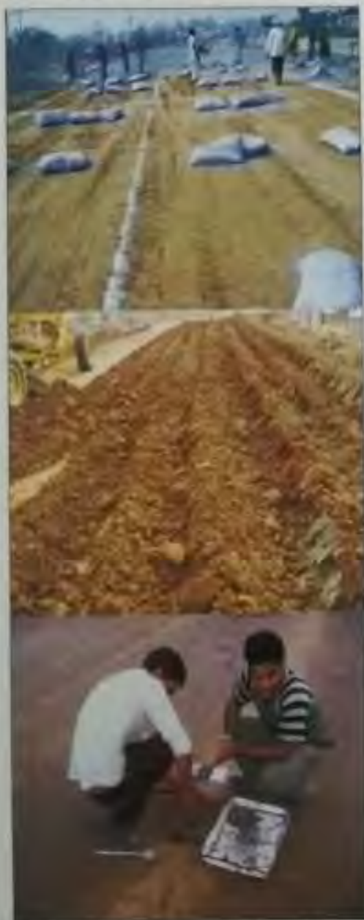
Fig. 6 Laying of cement, mixing of cement & in-situ density determination
