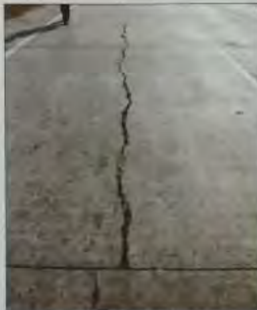
Fig. 56 Corner break crack
