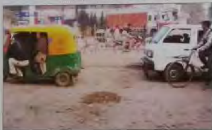
Fig. 58 A view of existing road
