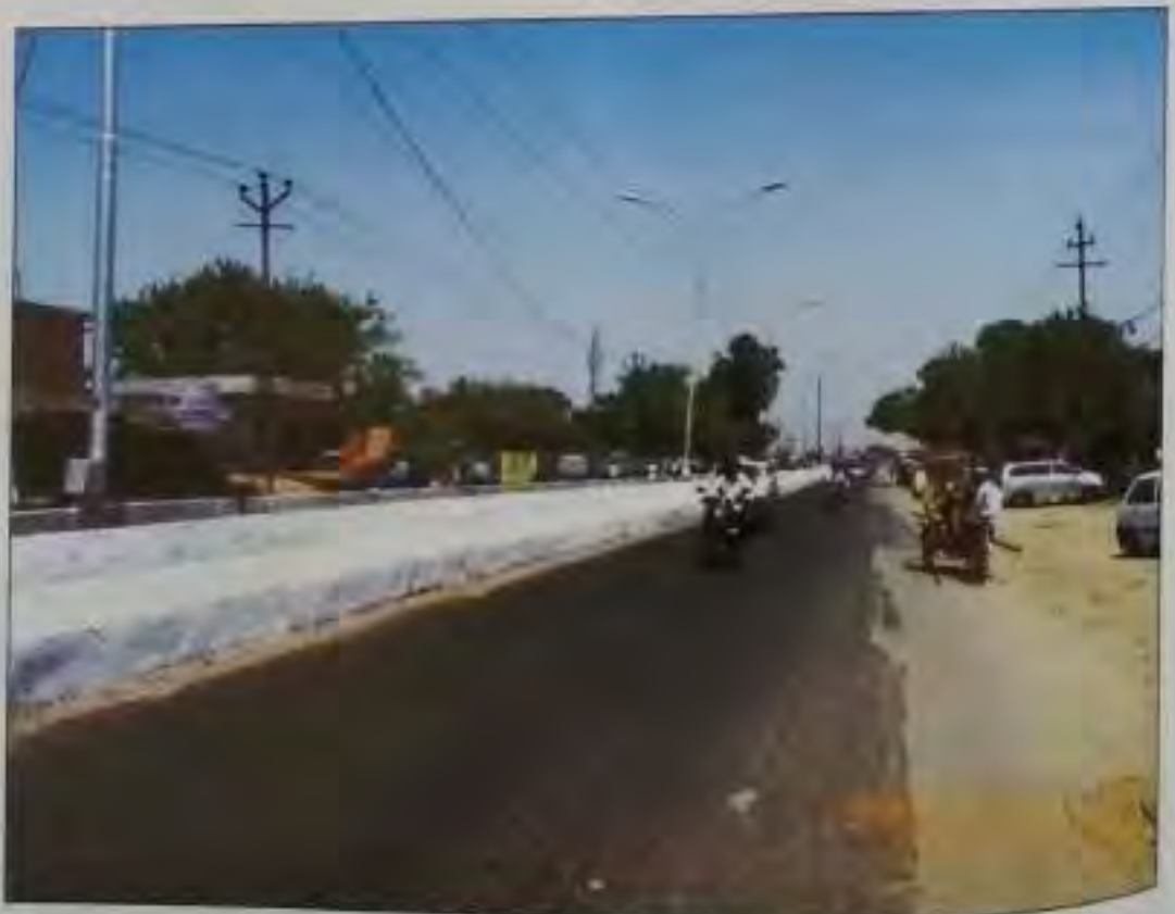
Fig. 63 A view of existing flexible pavement with profile correction course
