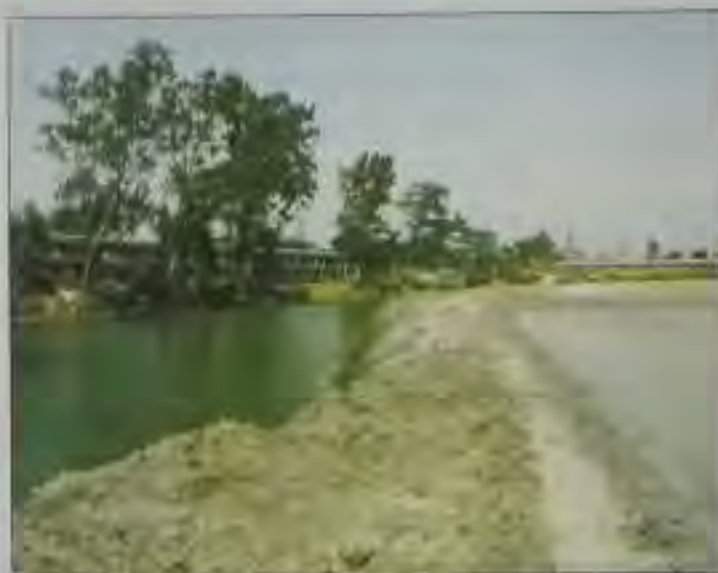
Fig. 28 Fly ash embankment construction in water logged area
