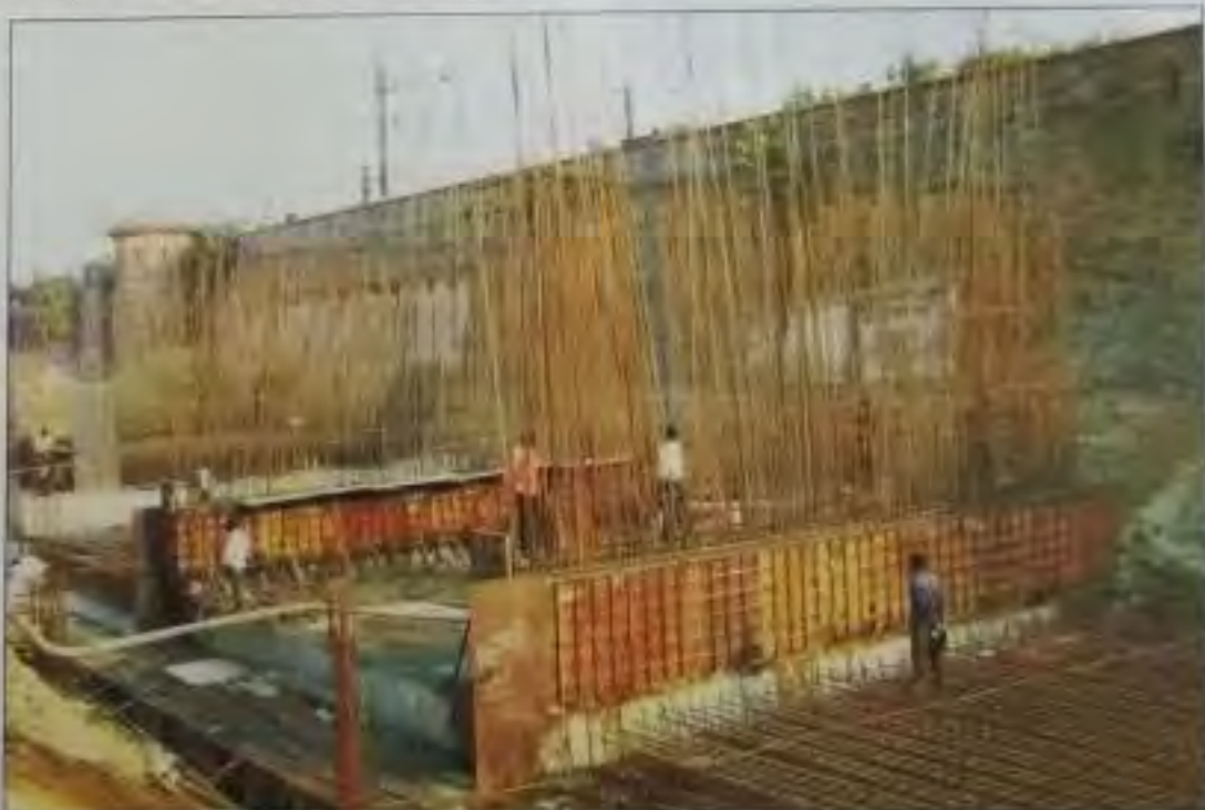
Fig. 10 Casting of RCC boxes after dismantling the retaining wall
