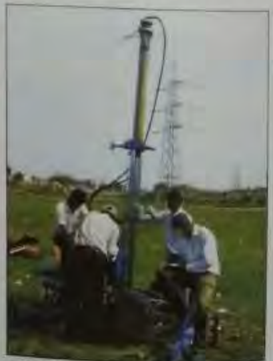
Fig. 26 SCP test being carried out at Signature bridge approach embankment site
