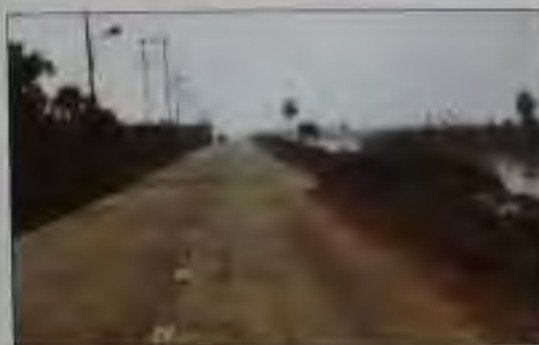
Fig. 62 A view of the constructed road
