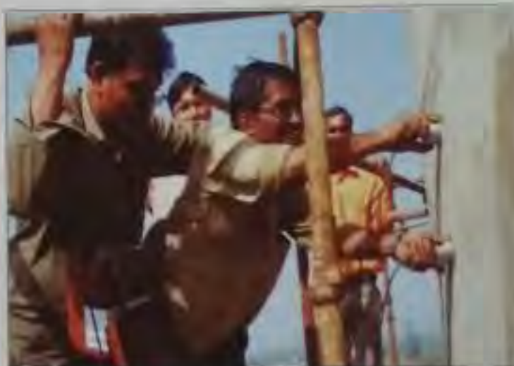
Fig. 94 Testing of PII of staging wall of the water tank at MBSQ
