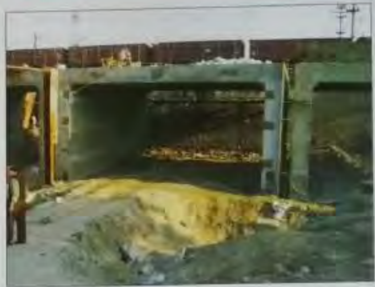
Fig. 9 - Boxes to be pushed inside the retaining wall
