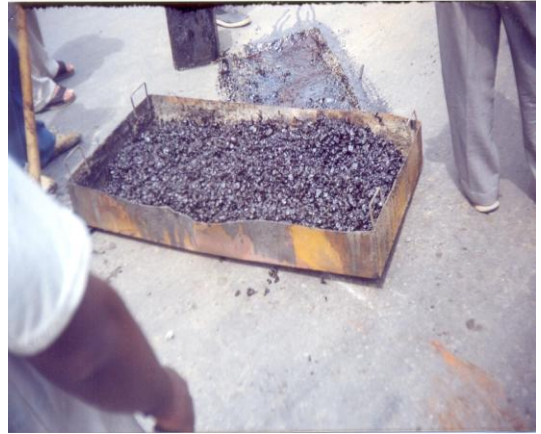
Preparation of cold mix with emulsion in tray in remote places
