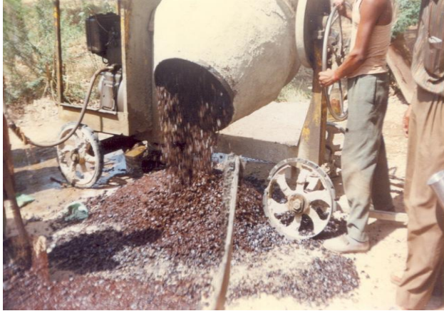
Preparation of cold mix with emulsion for stock piling the patching mix
