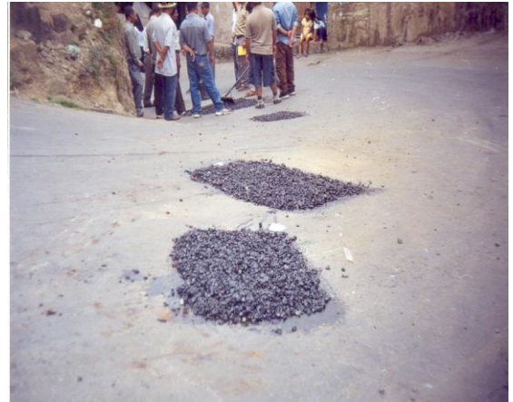
Preparation of cold mix with emulsion in tray in remote places
