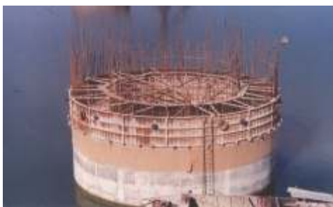
Instrumentation of Well Foundation at Ganga Bridge Varanasi
