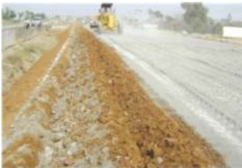
Soil stabilization with cement at Amritsar, Punjab
