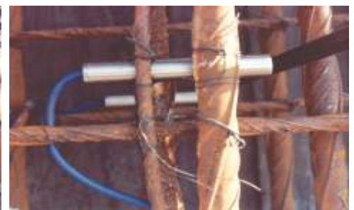
Installation of V W Temperature Sensor at Ganga Bridge, Varanasi
