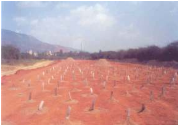
Ground improvement of marine soil with band drains
