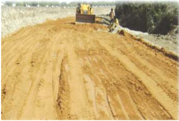
Construction of jarofix embankment, SH-9, Chittorgarh, Rajasthan
