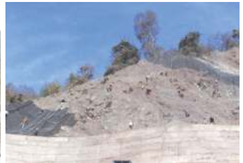
Remedial measures for Rock-fall at Zirakpur-Parwanoo expressway, Himachal Pradesh
